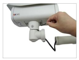
3. Push the excess length of cable through the ceiling bracket and align the ceiling bracket to the main bracket.
